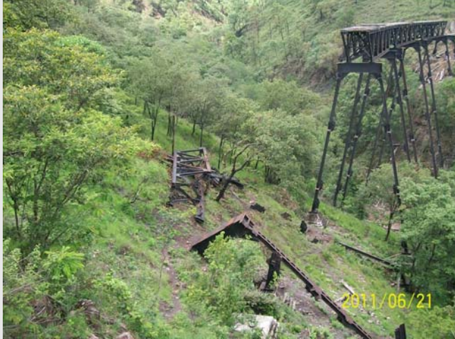
El Tecolote – mile post 181.53; photo by RDC
