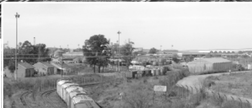
> On a busy day, ALL's Uruguaiiana mixed gauge yard is chock-a-block with freight cars awaiting transfer of goods and customs clearance. ALL Brazil has at least two EMD GL8 switchers working around the clock, one at each end of the yard. Notice that the yard is fully ballasted, to keep personnel out of harm's way during wet spells.
