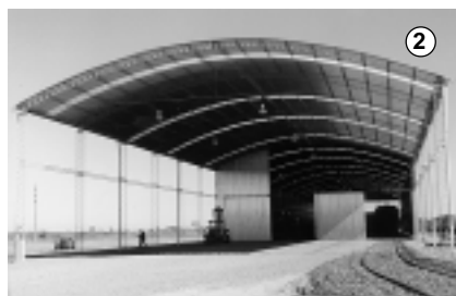
> (1-2) Westbound view of Zárate's intermodal terminal. The large shed, built at the yard's western end, facilitates cross docking and storage of paper products shipped by Alto Paraná, one of ALL Mesopotámica's major customers. (3) Zárate's intermodal terminal is equipped with a 50 ton rolling gantry. The 20-hectare facility was inaugurated in 2001. (J.C. González photo.)
