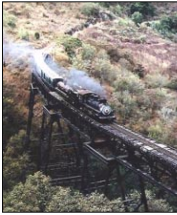
The poor state of bridge structures is a major worry.
