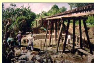
This bridge was rebuilt using 50 manual laborers and the highest technology was a cement mixer. The cost of the entire project – 200 miles of a national railway system, track, rolling stock, etc. – under US\$10 million. Why? Well, a railway with no revenue cannot justify an investment much higher than that.
