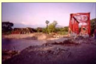
...after some creative engineering that included dragging the bridge (pictured above on its side) back into position using a bulldozer and a front-end loader (Truly a low technology approach!)
