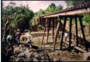
**1998 – Rehabilitation (cont.)...**This bridge was rebuilt with 50 manual laborers and a manually operated cement mixer.
