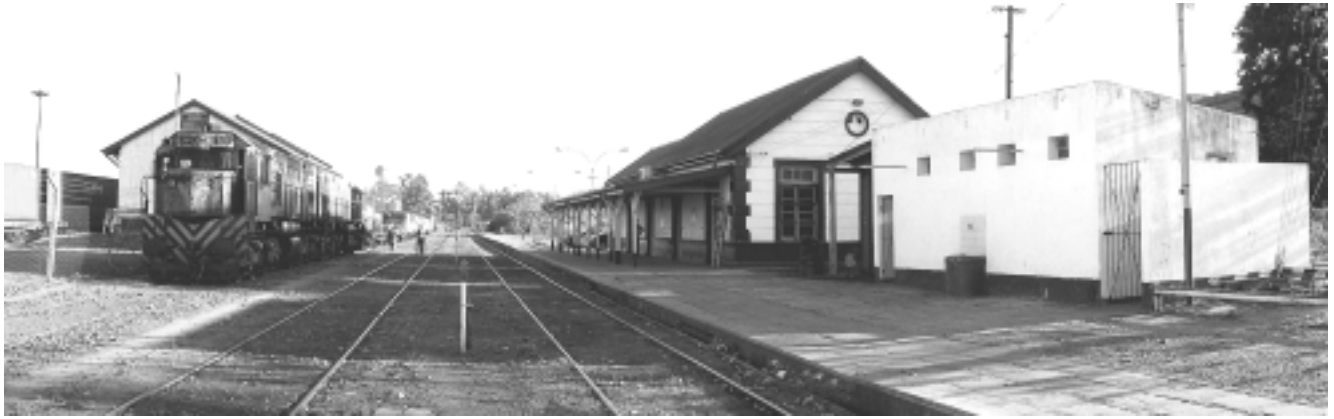
> Close-up view of Paso de los Libres station. The station building now officiates as Paso de los Libres Production Unit's main office. On the left, yard switchers GMIC G22s Nos. 7909 and 7925, working in multiple, are standing next to one of the station's freight sheds. This shed has been converted into a dormitory for crews and visiting staff.
